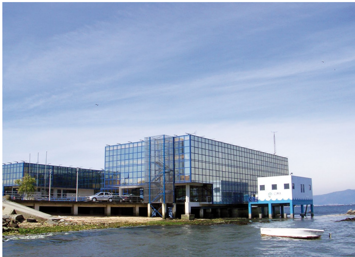
The CIMA headquarters in Pedras de Corón, Vilanova de Arousa (Pontevedra).
